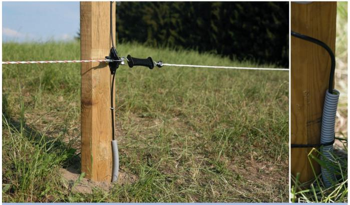
Tip: Underground cable must be laid in a plastic conduit to prevent damage to the cable!
